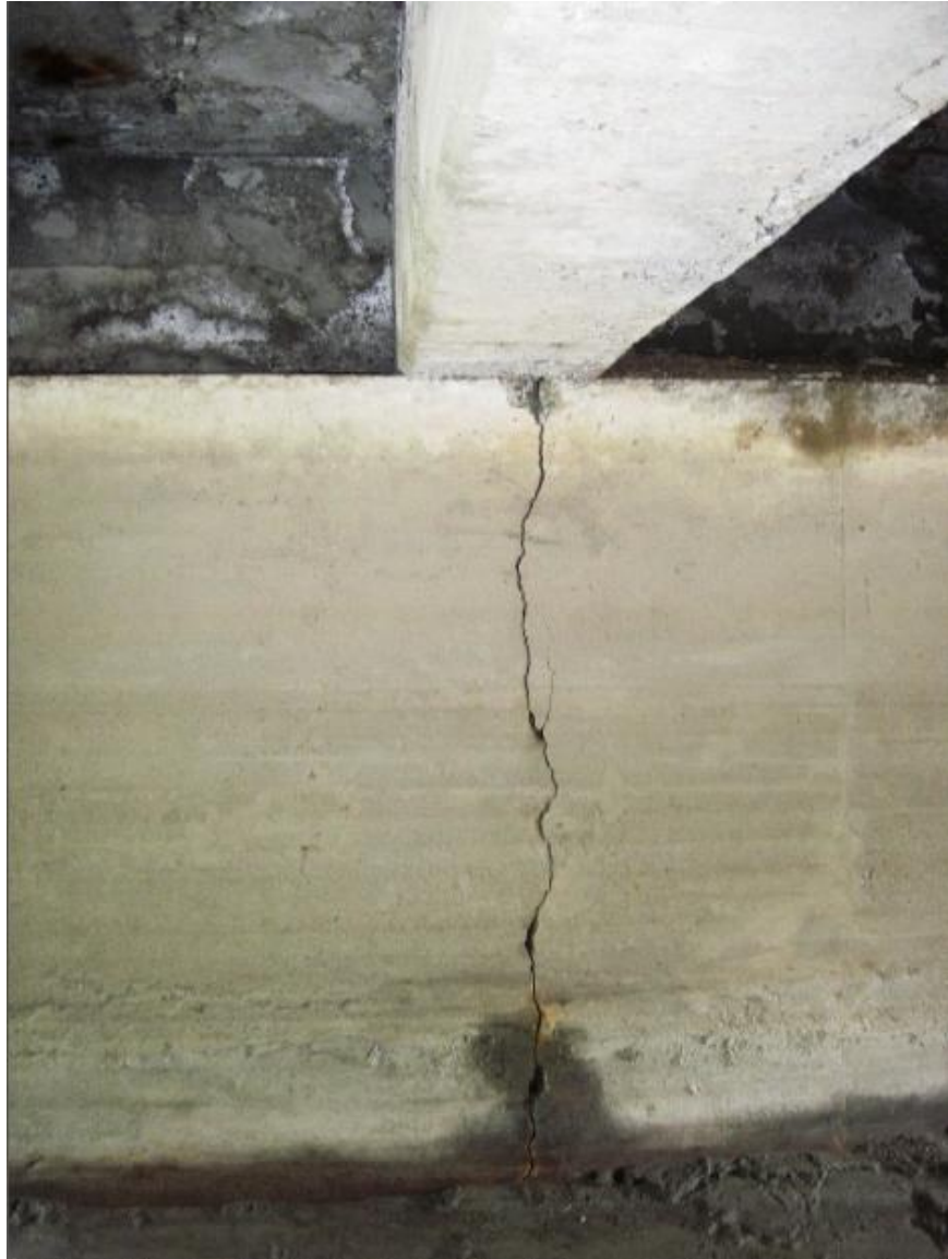
Vertical cracking in abutment.
