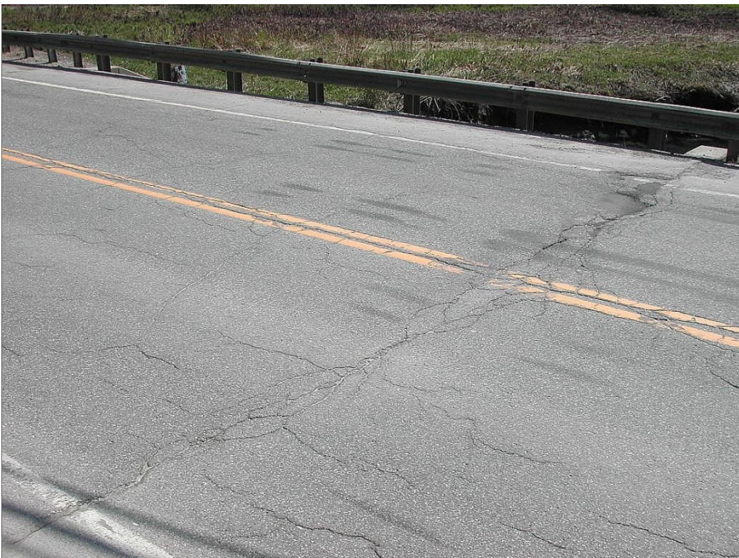
Deterioration and cracking along the deck.
