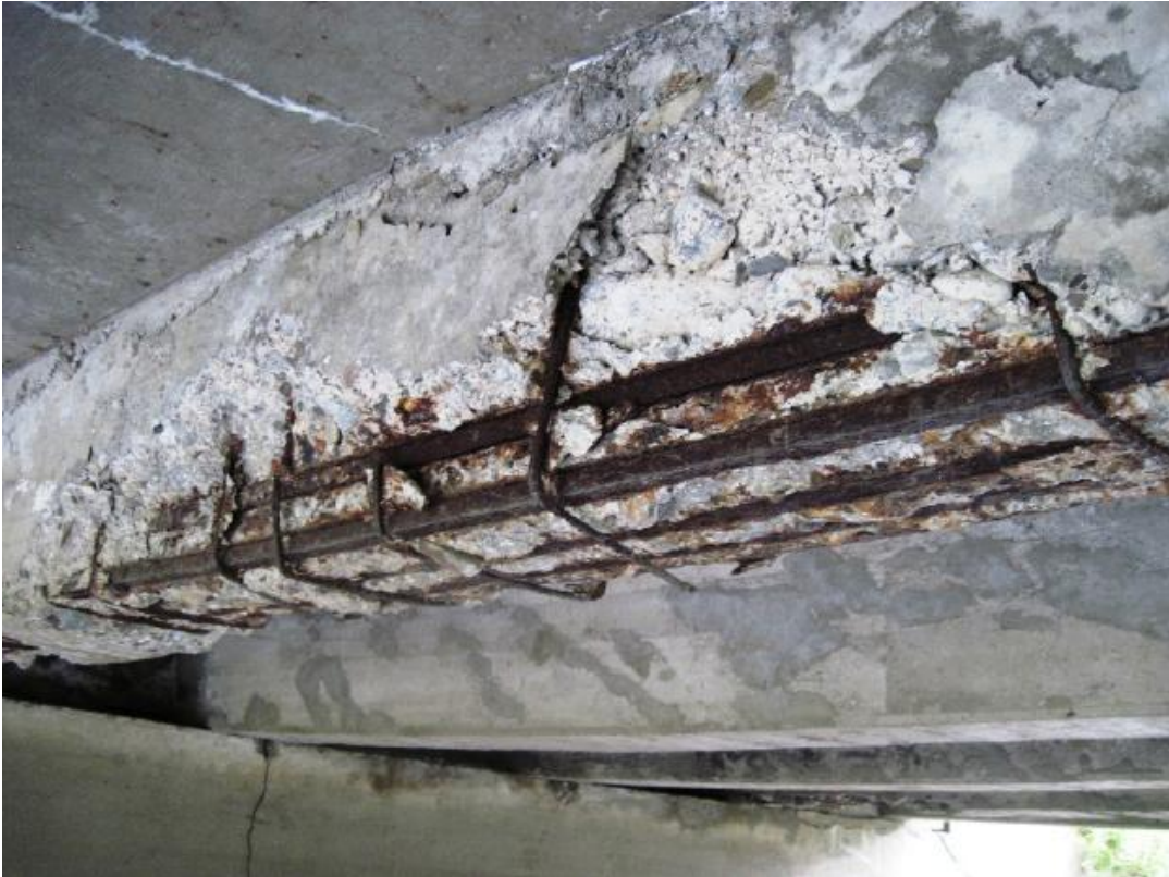
Deteriorated concrete and exposed rebar on the T-beam superstructure.
